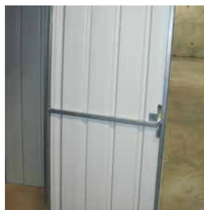
Upgrade to Steel Frame Door and Opening
